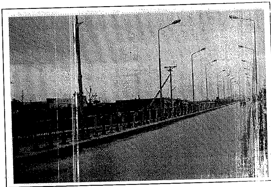
Figure 1. - General view of the bridge deck
